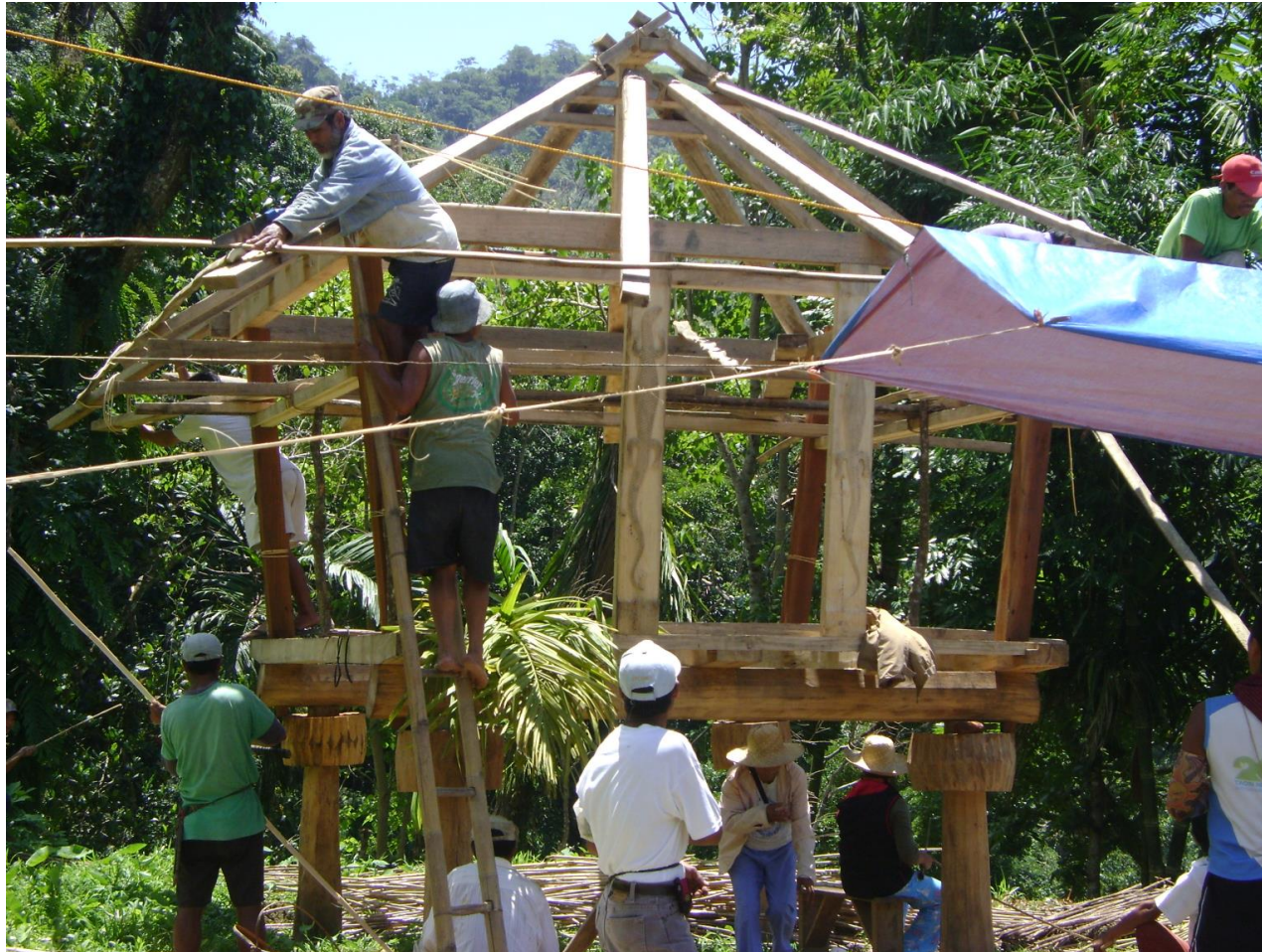
Figure 7. Construction of an Ifugao bale using local resources
